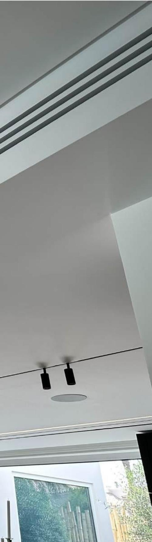
The Ventmann PERFORMANCE LINE vent diffuser combines elegant and adaptable design features with a specially engineered airflow that uses the Coanda effect, making it ideal for air conditioning. This is a model that empowers you to craft distinctive interior features or seamlessly conceal the diffusers, while minimizing direct airflow onto users.
